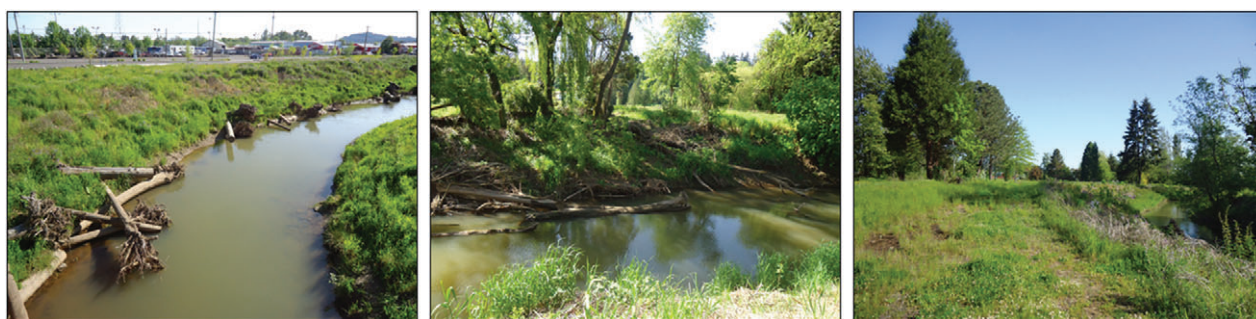
Figure 2 East Lents floodplain restoration.
